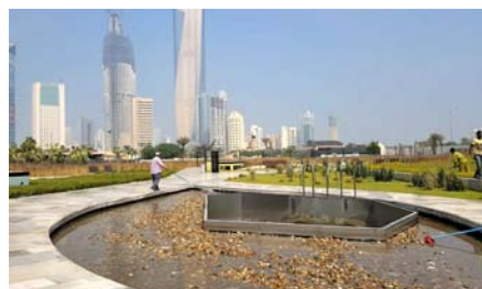
Stabilodrain® elements applied on the approximately 15,000 m 2 of ceiling surface of the underground parking provide a stable base for green areas, paths and seating. Gaps in the water basin allow for natural illumination of the garage and water features provide cooling.
